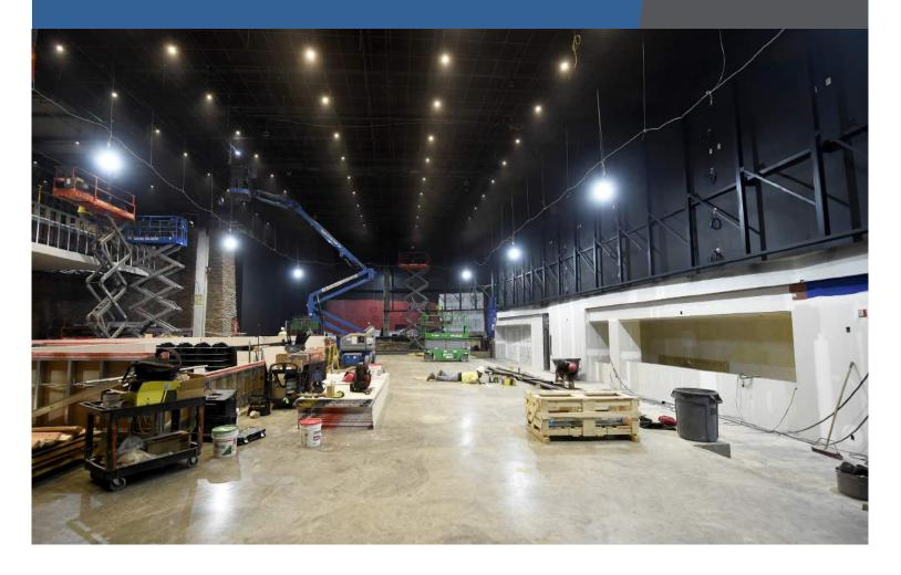
After the steel structure was in place, the SEAMLESS Bespoke Mounting System was installed, and the displays were mounted row by row so the whole video wall came together easily and flawlessly. The team included a half-inch vertical expansion gap between each of the sections to account for a potential difference between snow loading deflection that could impact the side sections of the curved video wall differently than the main wall.
