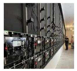
The 256 LG cabinets (1,024 modules) were shipped in 32 crates and each cabinet was labeled for its exact location on the wall, which took a lot of methodical organization when unboxing. The cabinets are cableless, with all power cascaded from one cabinet to the next. The 65/35 heat ratio allows install into shallow recessed cavities. From a servicing standpoint, everything can be serviced, maintained, or swapped out from the front.
